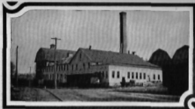
SHEFFIELD FARMS-SLAWSON DECKER PLANT
