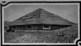
AT THE SEWAGE DISPOSAL PLANT
