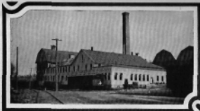
SHEFFIELD FARMS-SLAWSON-DECKER PLANT
